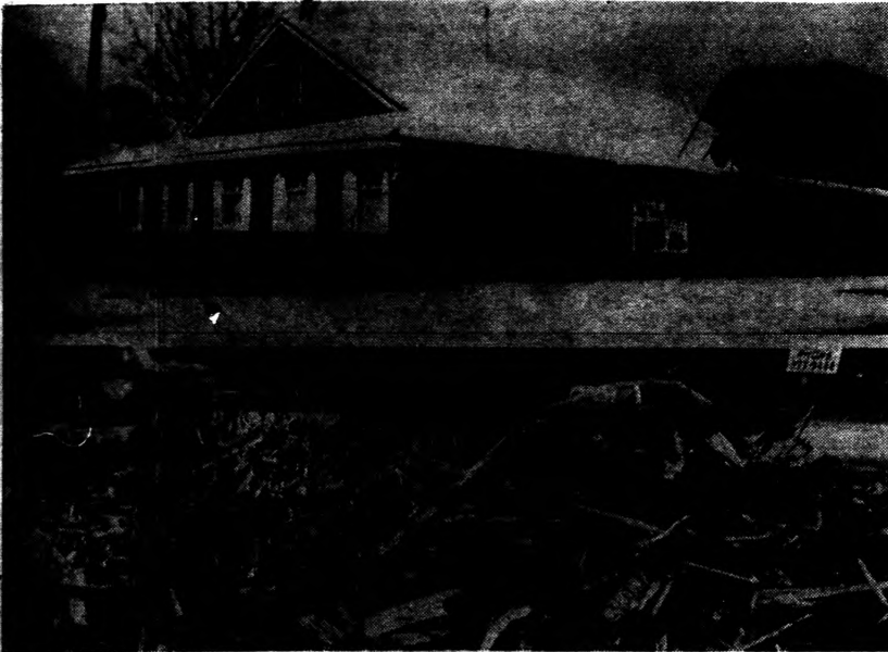
DISAPPEARING ACT — Only a pile of rubble remains of Dan Dowd's Steak House on Route 23 South. The restaurant was a well known area landmark for many years but was vacant for several years. It is making way for urban renewal and is one of five buildings razed so far. Pictured above are before and after photos.
