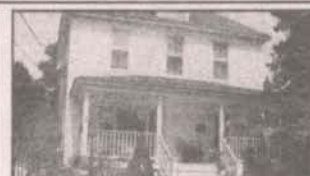
POMPTON LAKES $429,900 Lemonade Porch Colonial! 3 BRs, 1.5 Baths, newer roof siding, doors. Baths, full walk-out bsmt. Garage with loft.
