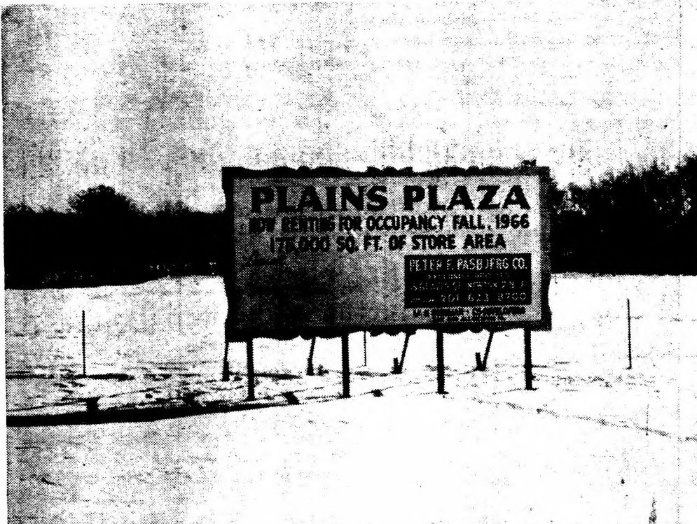
NOW RENTING — A large sign, denoting the fact that stores will be available in the giant Grant City shopping complex, to be known formally as Plains Plaza, was posted on the site last week. Including the Grant store, the shopping center will offer 175,000 square feet of store area. The site is at the Pompton Plains traffic circle on Route 23.
